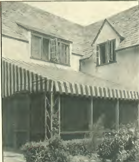
(Left)—An out-door living room has been made of this terrace. Screens extend to awning and porch may be completely dismantled in winter.
